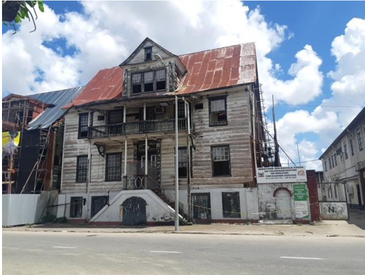
Upper: before renovation. Photo credit: Daily Krijnen (2023)
